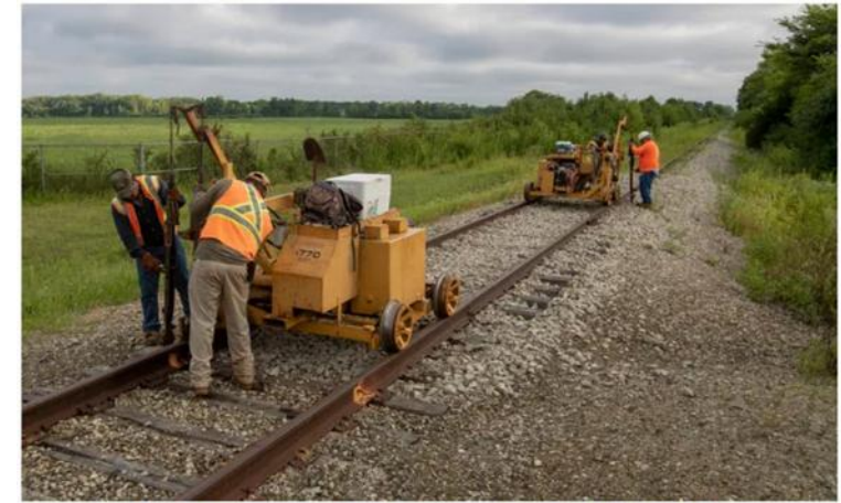
A crew for Utah's A & K Railroad Materials removes railroad spikes Wednesday on the Nickel Plate Line. Robert Scheer
